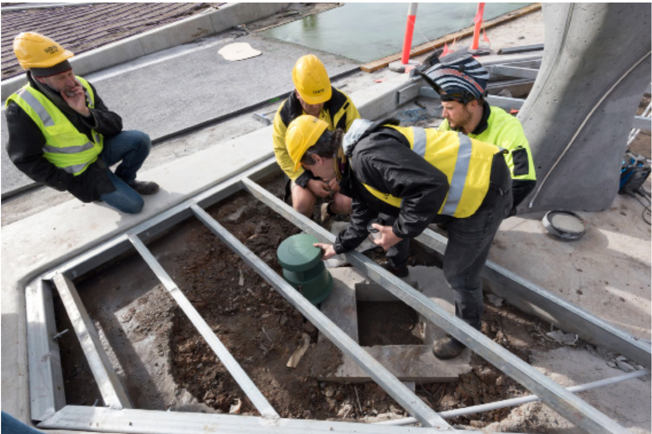
Figure 5. Installing and securing the in-ground speakers. Courtesy of Chuan Khoo
