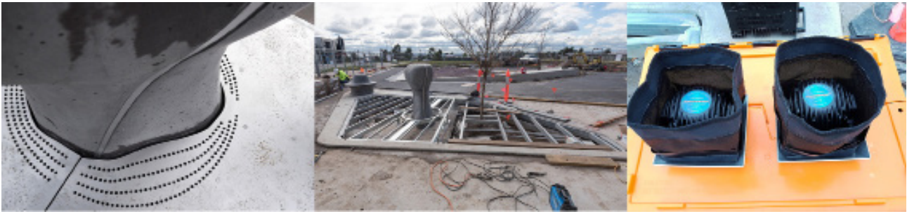
Figure 4. The central image shows the two transducer beams stretching away from the sensing stone. A water-proofing solution for the transducers (right) was created before being attached to the transducer beams. The left image shows the concentric contours of stone and plate, which allows for uplighting effects. Courtesy of Jordan Lacey
